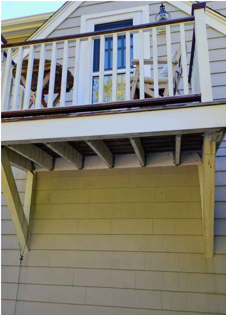
Balcony off Guest Room/Office
